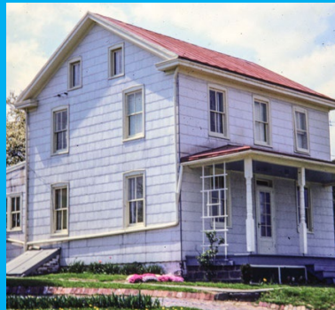
The family house at RR #1 Willow Street
